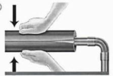
Close the slit seam and squeeze together with firm pressure, to ensure a permanent seal.
