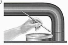
Seal All joints with Armaflex Adhesive. Do not stretch when sealing joints.
